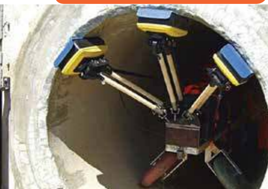
Non-destructive pipe scanning
